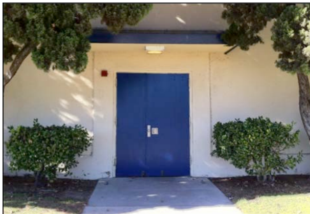
Figures 48. and 49. If ADA-compliant access cannot be accommodated at primary entrance without damage to character-defining features, consider using the California Historical Building Code and its alternatives for ADA-compliant access on secondary entrances. Install ADA-accessible ramps in a way that allows for ease of access while also limiting visual obstruction of important character-defining spaces and features to the maximum extent feasible. Source: LAUSD, 2014.
