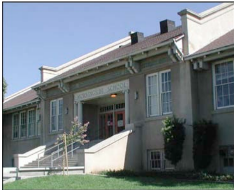
Figures 11. and 12. Roof brackets and exposed rafter tails, Morningside Elementary School (1915, left). Wide, unadorned cantilevered eaves, Leapwood Elementary School (1962, right). Source: LAUSD.
