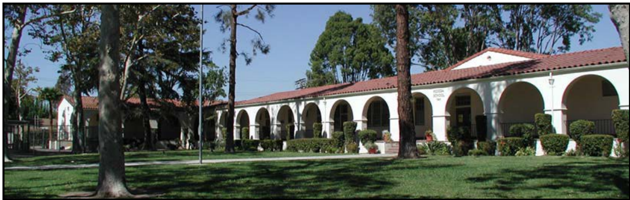
Figure 65. Reseda Elementary School, 1936. The spare Mission Revival style was in keeping with the post-Field Act requirement for one-story massing and the post-Long Beach Earthquake trend to design in the “traditional Southern Californian” mode. Source: LAUSD.
