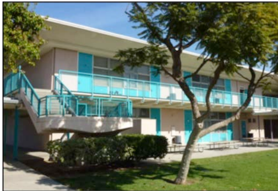
Figures 11. and 12. Roof brackets and exposed rafter tails, Morningside Elementary School (1915, left). Wide, unadorned cantilevered eaves, Leapwood Elementary School (1962, right). Source: LAUSD.
