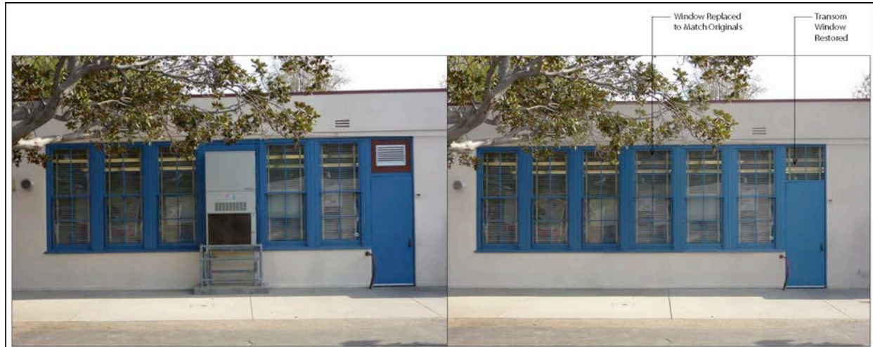
Figures 46. and 47. Where possible, removing inoperable HVAC units and restoring windows to match originals enhances the appearance of historically significant LAUSD buildings. Source: LAUSD and Architectural Resources Group, 2014.
