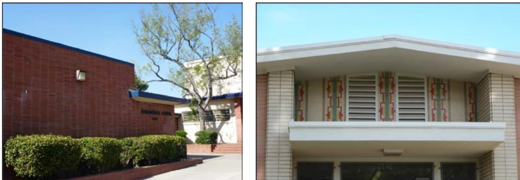
Figures 7. and 8. Mid-Century Modern details: stack-bond brick veneer, Fernangeles Elementary School (left), and patterned tile at classroom entries, Chatsworth High School (right). Source: LAUSD, 2014.
