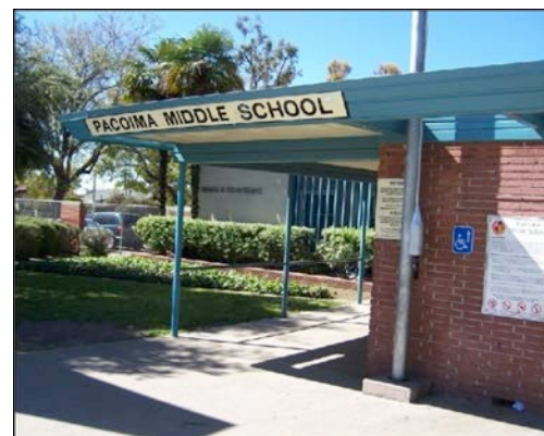
Figure 104. Pacoima Middle School, Administrative Building (1955), Wilmington. Source: LAUSD Pacoima Middle School Pre-Planning Survey, 2010.
