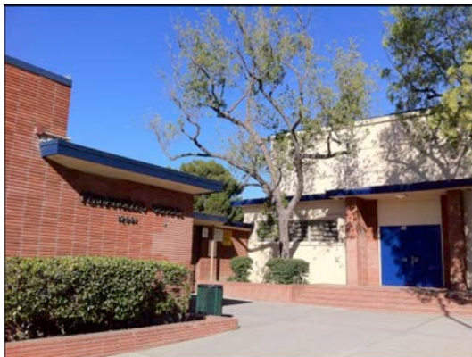
Figures 15. and 16. Mid-Century Modern roof treatments: flat roof with no eaves combined with cantilevered projections, Fernangeles Elementary School (left) and roof cut-out/skylight at Castle Heights Elementary School (1951, right). Source: LAUSD, 2014.
