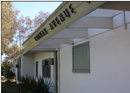
Figures 13. and 14. Modernist roof treatments: extended, trellis-like eaves, Colfax Avenue Elementary School (1950, left). Zig-zag roofline, Palisades High School (1963, right). Source: LAUSD, 2014 (left), SWCA Environmental Consultants (right).
